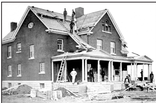
Construction of Bismarck's Fort Lincoln began in 1900
